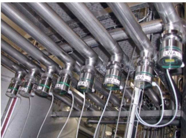
**Conductivity measuring units ILM-2** in the CIP return line for the separation of cleaning media. One unit for each CIP cycle. Depending on the conductivity, the medium in the piping is recognised and directed back into the correct CIP vessel.
