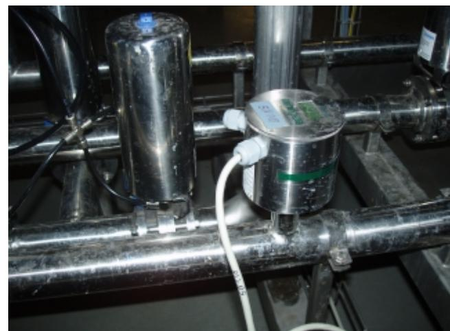
**Turbidity measuring unit ITM-2** for phase separation milk - water. Used during emptying of a production plant. After completion of production, the plant is flushed empty with water. With the ITM-2, it is exactly determined when the plant is fully and thoroughly emptied.
