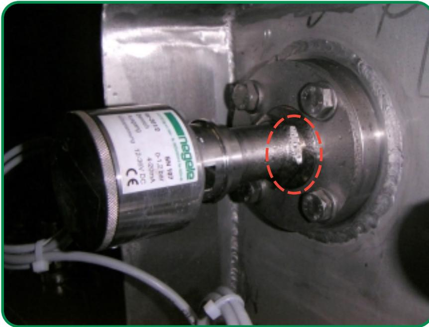
**Pic. 1: Condensation at the level sensor LAR-361**
