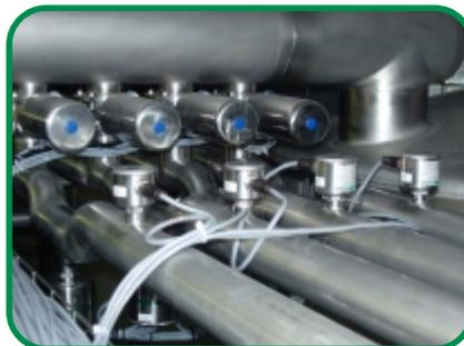
**Fig. 3: Flow monitor, type FWA-141, built into the return for monitoring the CIP circuit.**
